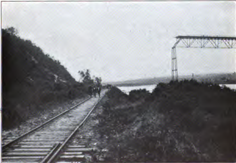
FIG. 2.—SMITH AVE. VIADUCT. LOOKING UP STREAM. SHOWING SECTION OF VIADUCT THROWN DOWN BY STORM.
